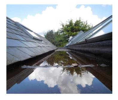
The secret box gutters to each side of the atrium have been constructed with inadequate falls, with virtually no upstand to either side of the gutter. The outlets are inadequate to cope with the volume of water discharging from the adjacent roofs into the secret box gutters and therefore, under periods of heavy rainfall, the gutters flood up over the inadequate upstands and the water tracks into the property. The image to the left shows the lack of fall and ponding of the gutters.
