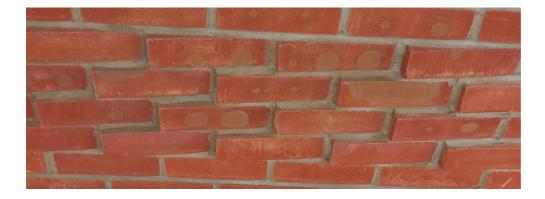
Where the proposed projecting bricks include frogs or perforations, this can have a negative impact upon the integrity and thus durability of the brick, potentially reducing the service life of the brick below the required 60 years as required by our warranty.
