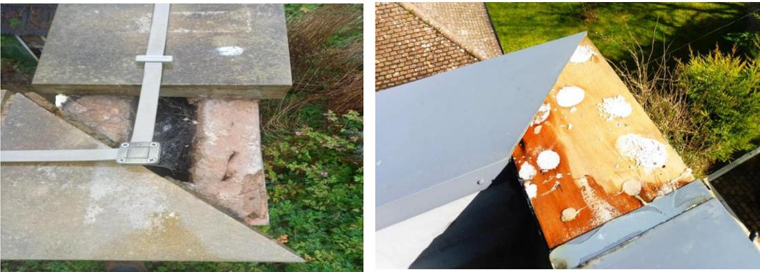
Image top left represents a situation where the DPC and DPC support has been omitted. As a result mortar bedding is not present and the coping has detached. Image top right represents a situation where the DPC has been omitted and the capping has been attached using mastic. Adhesion has failed and the lack of mechanical fixing has resulted in detachment and water ingress.
