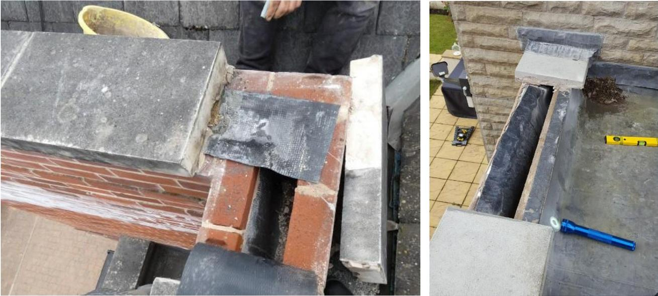
Failures in the horizontal DPC are common place. In the image to the left, we can identify a DPC of incorrect width, a lack of support to the DPC as it crosses the cavity and a lack of sealed joints in the DPC. The image to right shows a complete omission of the DPC, which has compounded the cavity tray issue (described below).
