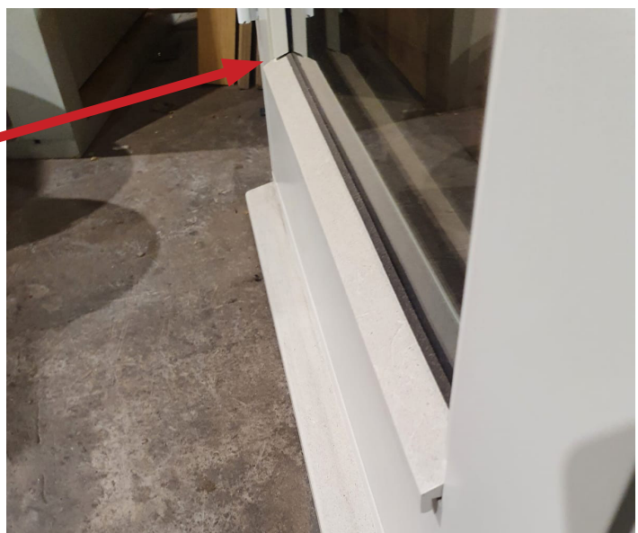
Image showing correctly scribed beading
